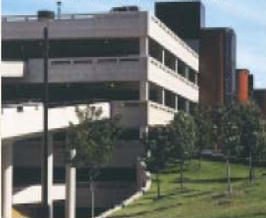
Baltimore-Washington International Airport Parking Structure.
