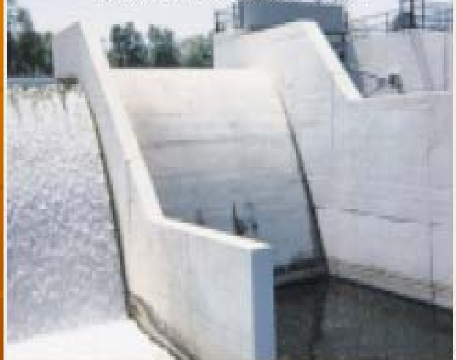
Mass Concrete: Sylvan Lake Dam, stilling basin, Rome City, IN
